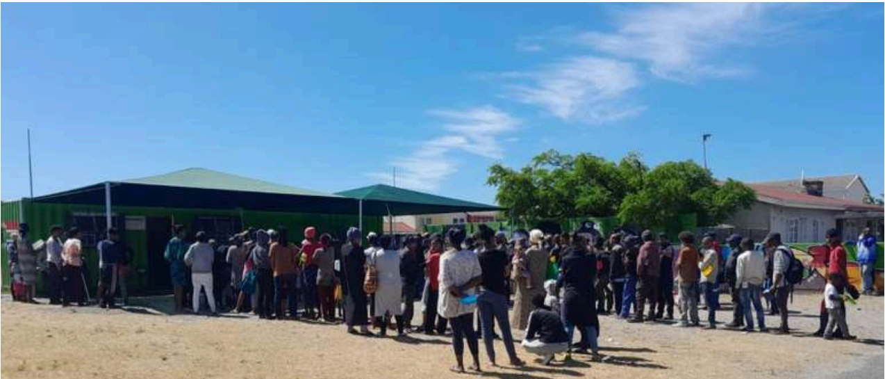
The new shade port providing shade to people waiting in line at the feeding scheme
